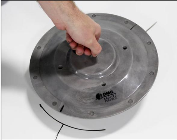
**STEP 7:** Using the bolts supplied, hand tighten all four bolts to secure the cover plate to the base plate. Once hand tightened, use a ratchet to tighten bolts. Bolts should be applied at a torque of 60-70 in-lbs.
