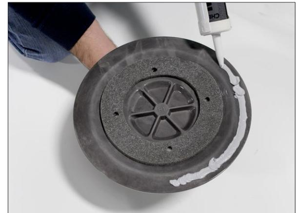
**STEP 6:** Lay cover plate onto base plate, taking care to align it using the indicator marks made in Step 4.
