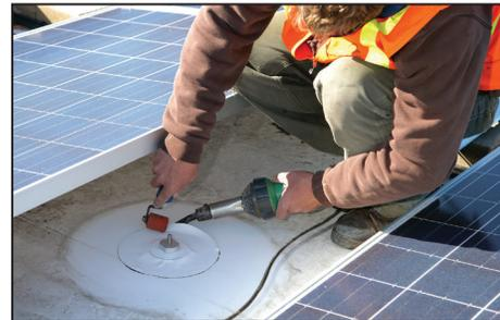
**Figure 3:** These roof mounts are heat welded in place to ensure that they too remain watertight.
