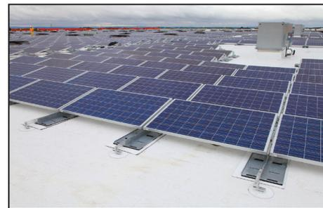
**Figure 4:** Mechanical roof mounts not only reduce rack movement on the roof, but can also eliminate the need for ballast.
