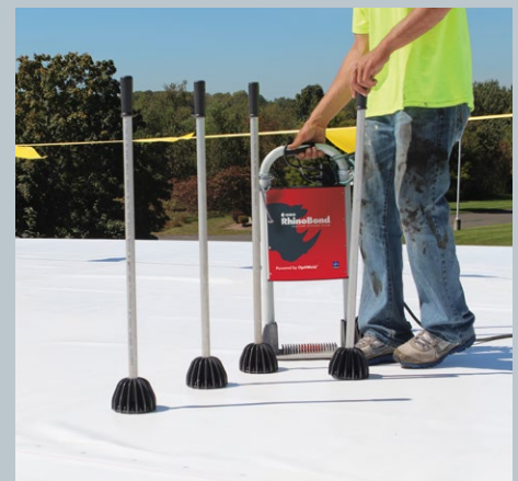
3. After the membrane is installed, weld each plate using the RhinoBond tool.
